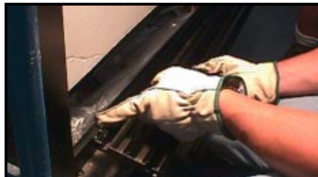
Figure 50 - Place Control Access Panel
